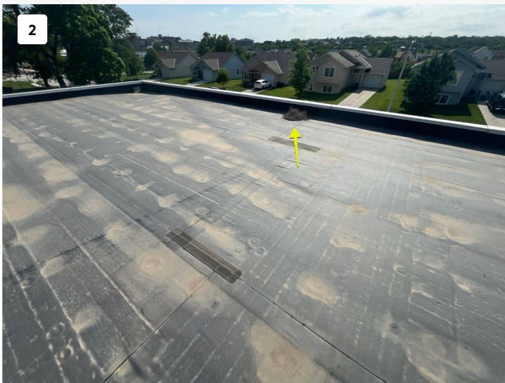
Minor detail patching has been performed.
