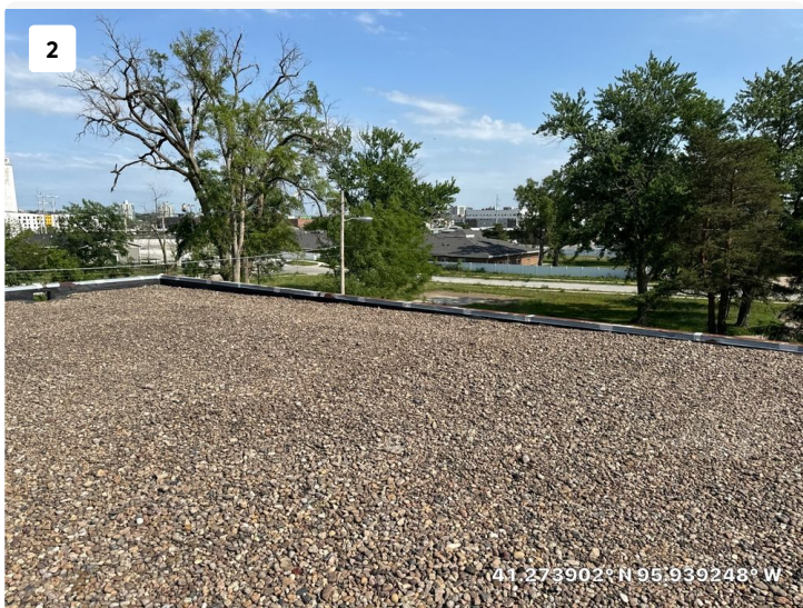
Rock coverage is great. No gaps in coverage.
